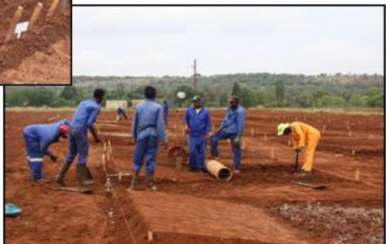
Figure 7. Compaction of the runoff collection areas of the in-field rainwater harvesting and conservation technique at Roodeplaat, ARC-VIMP.
