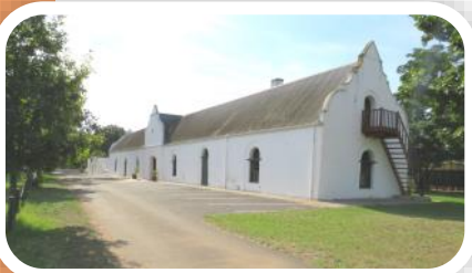
The current admin building
