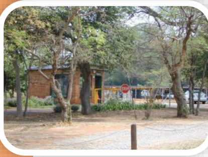
The security house and boom at the Rietondale farm
