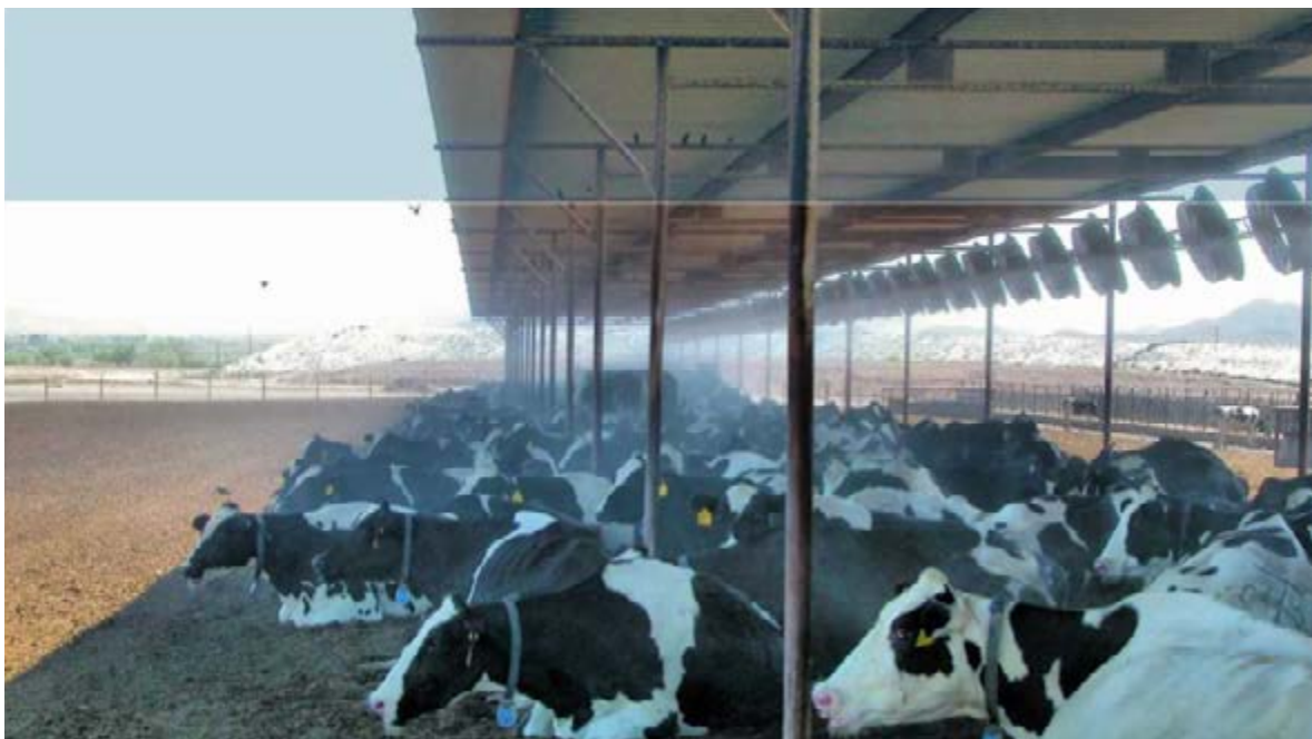
Figure 10 Sprinkler and fan cooling.
