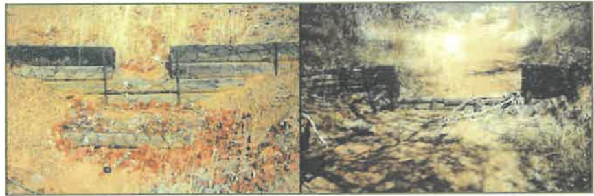
Figure 3: Typical permeable timber pole structures.
