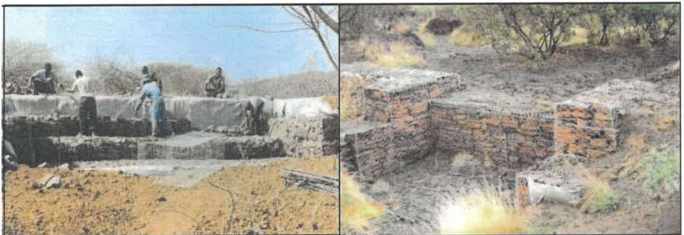
Figure 3. Typical gabion retaining structures
