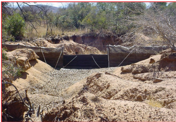
Figure 3: A finished silt fence.
